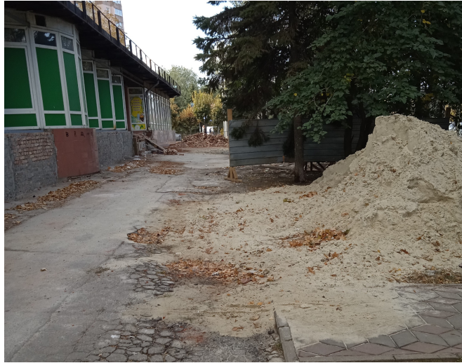
Construction next to the Church building
